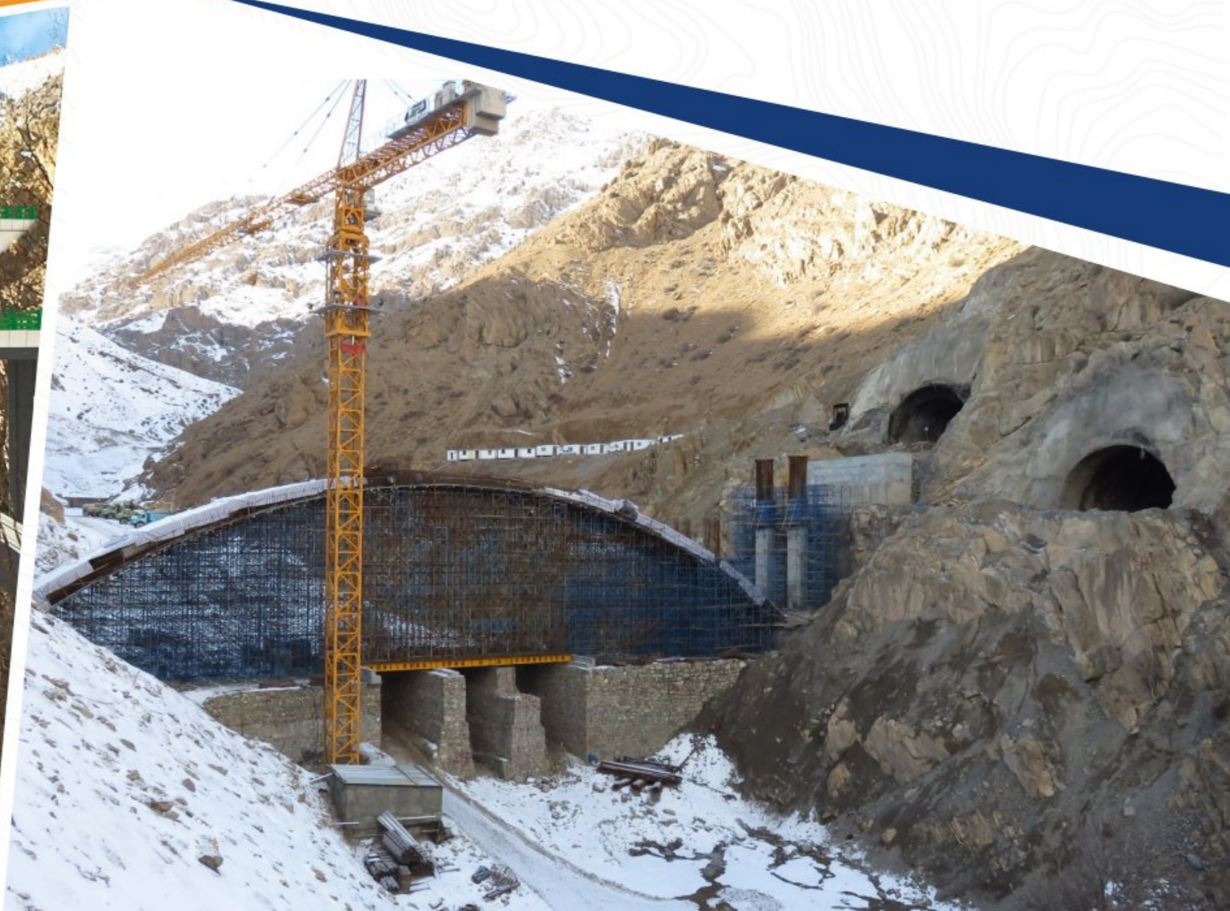
Hasanakdar Arched Bridge (Tehran- Shomal freeway)
